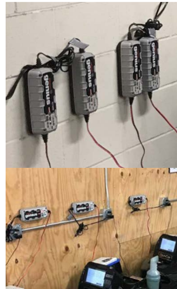
Figure 15 Examples of Charger Mounting Orientation
